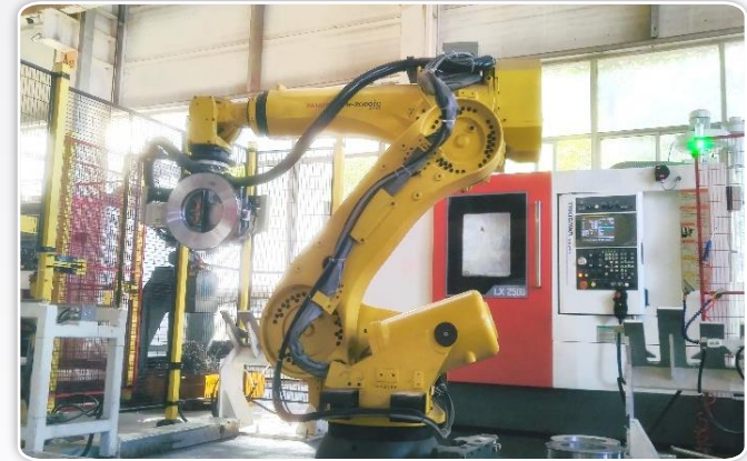
CNC machining process line
