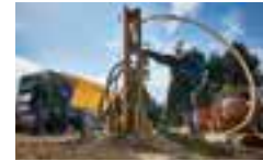
14 bar: blast hole drilling or ground engineering drilling
