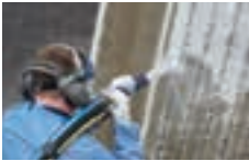
8.6 to 10 bar: Abrasive blasting
