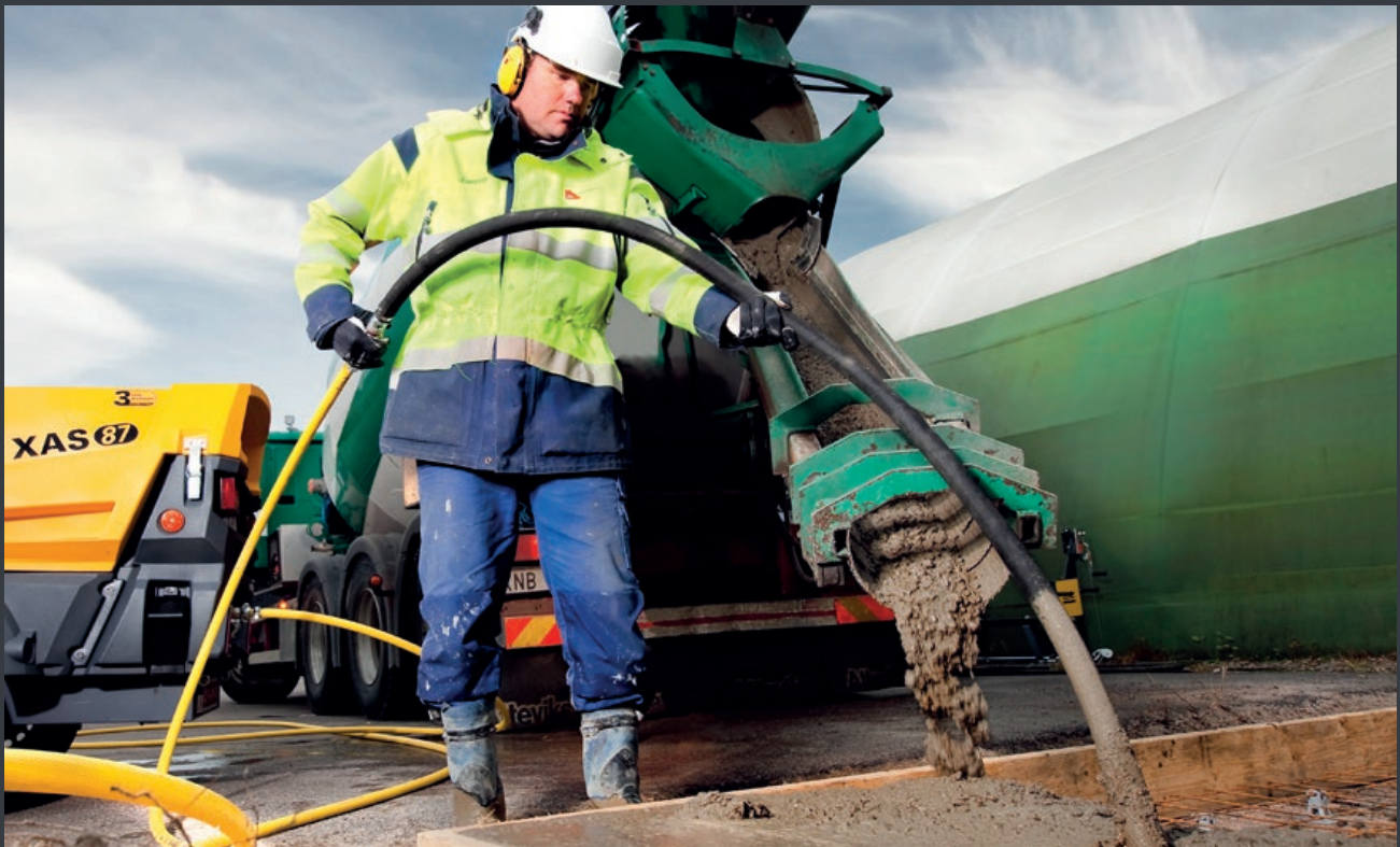
One of the advantages of pneumatics is that the air keeps the temperature of the pocker head down.
